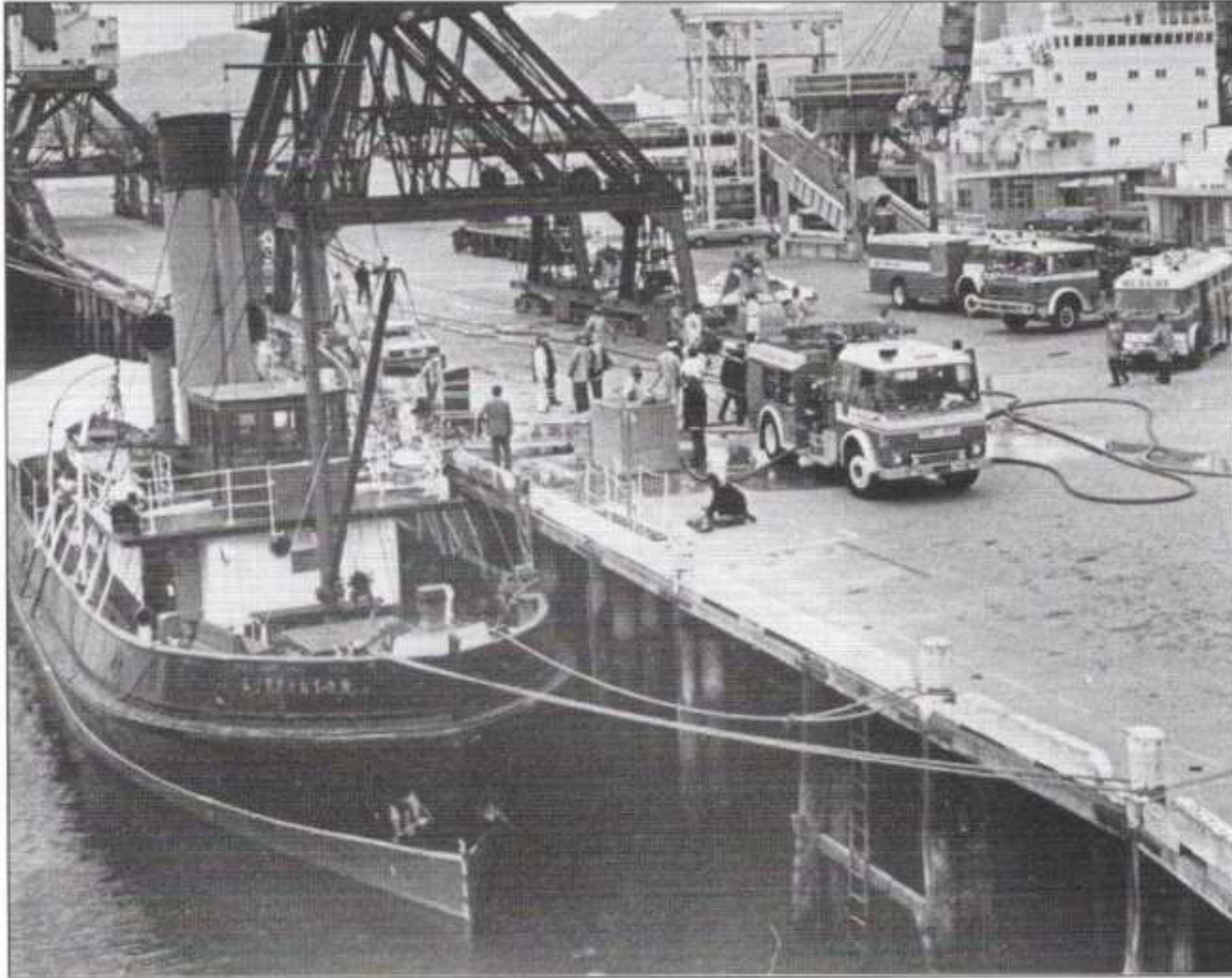
Anxiety in December 1984, as fire engines attend a fortunately minor fire in the coal in the port bunker.
