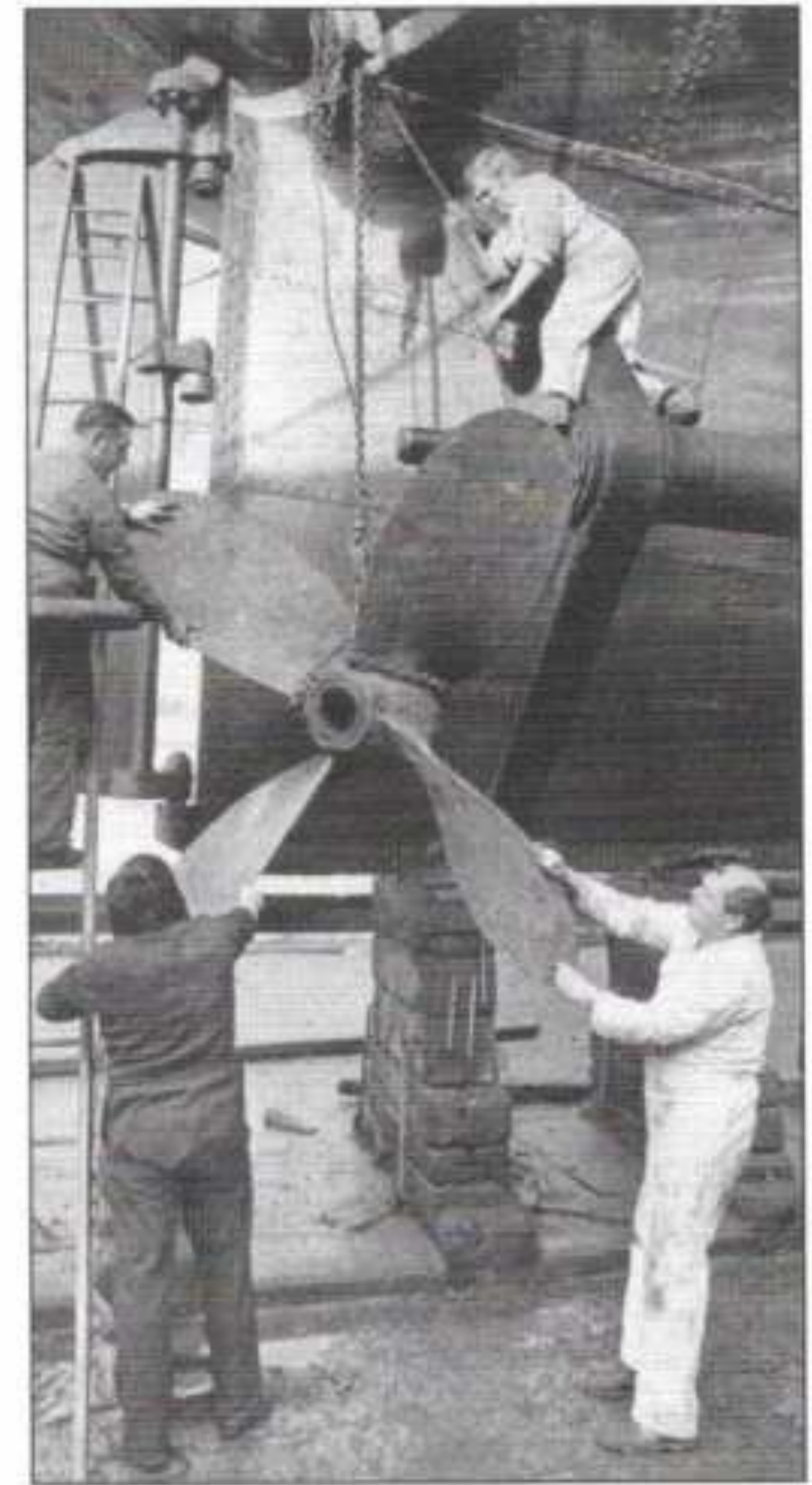
June 1973 – members of the newly-formed tug society remove the starboard prop for the shaft to be drawn. Bill Le Warne junior (top right), Bill Le Warne senior (lower right), and Bill White (top left). THE STAR
